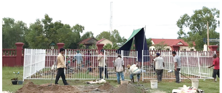
▲ Civil works to construct a foundation, 2020
