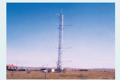
• Dust storm monitoring towers at Duolun in the source region
