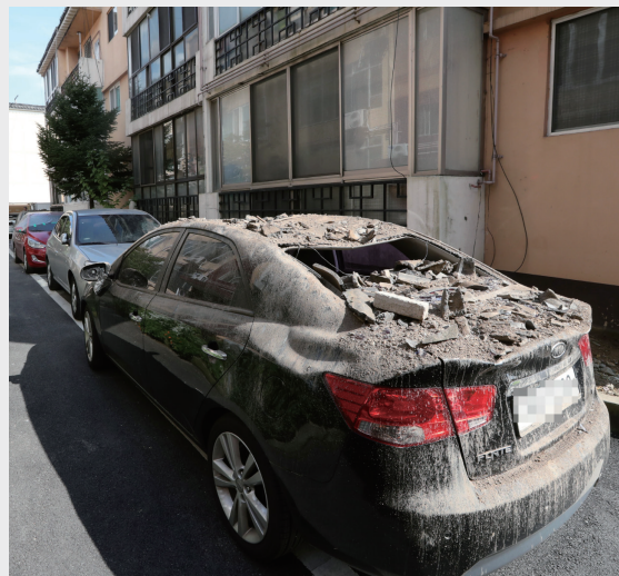
The earthquake damage in Gyeongju
